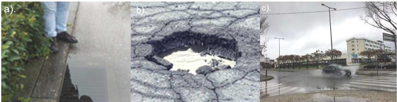
Fig. 1. The effects of the heavy rainfall on the roads, Ave. Universidade de Aveiro, Aveiro, Portugal: a). Overflow from the urban drainage with limited capacity in critical rainfall conditions. b). Effects of inefficient drainage on the streets. c). Traffic disturbance and crossing problems caused by the insufficient urban drainage capacity in critical rainfall conditions.
