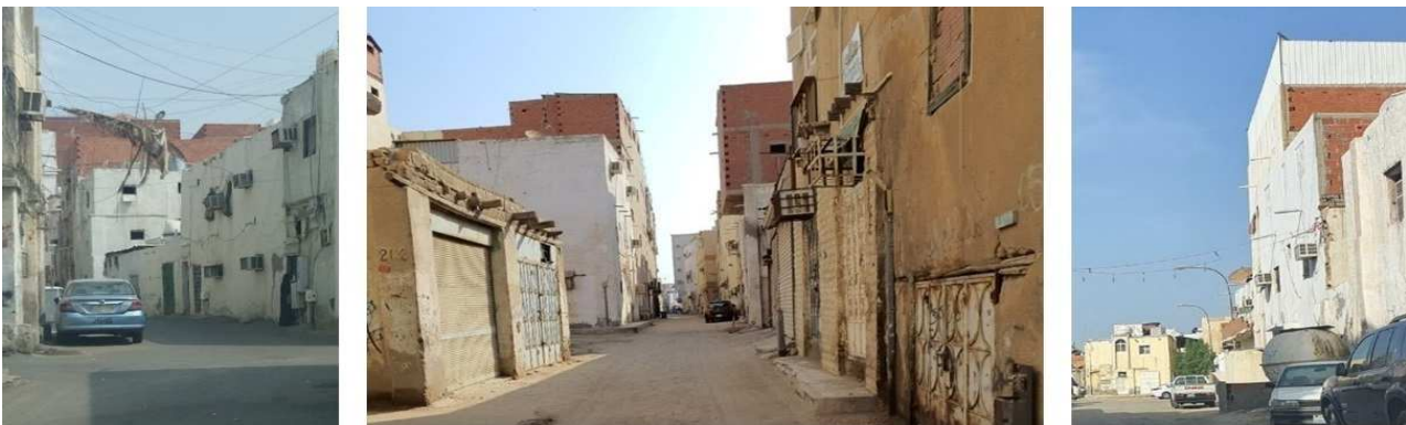
Fig. 8. Buildings of different heights in Al-Sabeel District.
