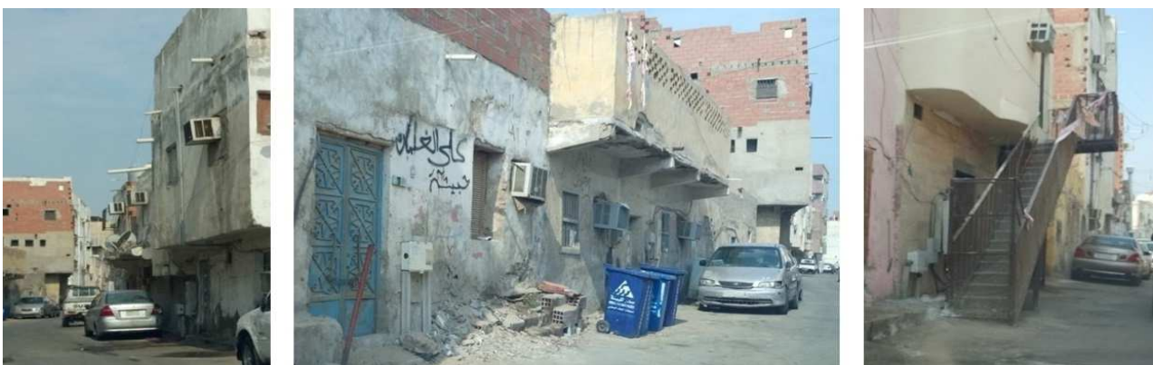
Fig. 9. Construction materials used for buildings in Al-Sabeel District.
