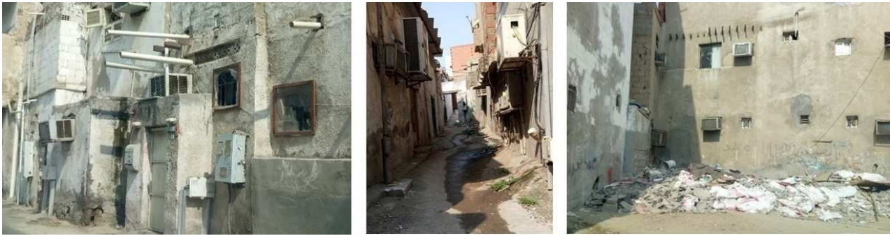
Fig. 10. Deteriorated infrastructure, exposed electrical wires, sewage, uncollected rubbish.
