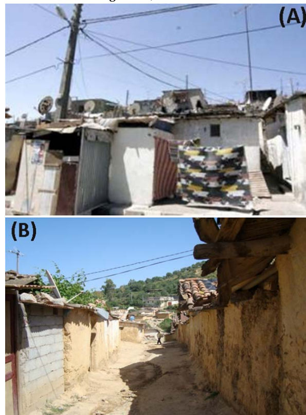
Fig. 3. Types of precarious housing. Slums of Algeria 2010 (A), and houses of the colonial period (B).
