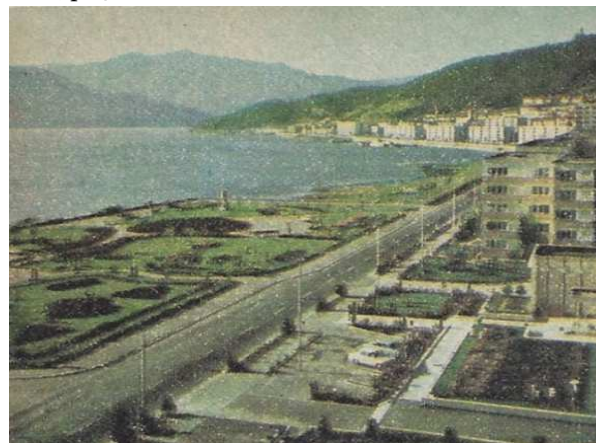
Fig. 3. Amorphous mass-housing in new Orșova: “The new town Orșova” (source: Iancu, Motrescu and Negulescu, 1985, p. 47).
