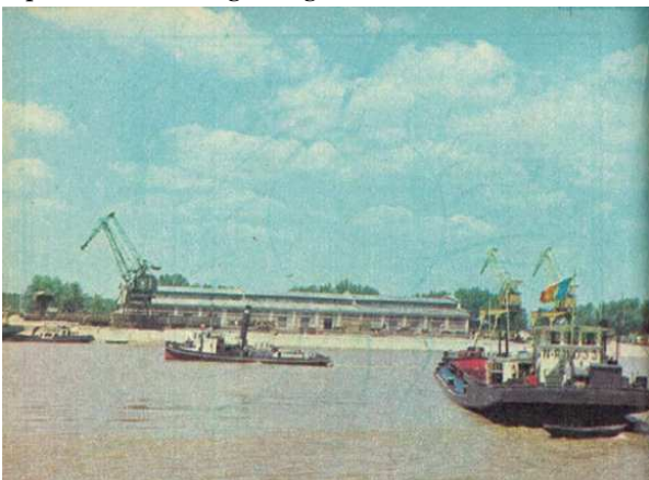
Fig. 11. Massive redevelopment of Giurgiu: “The Danube at Giurgiu” (source: Giurcăneanu, Mușat and Ghica, 1986, p. 64 ).
