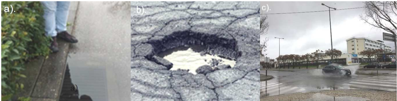
Fig. 1. The effects of the heavy rainfall on the roads, Ave. Universidade de Aveiro, Aveiro, Portugal: a). Overflow from the urban drainage with limited capacity in critical rainfall conditions. b). Effects of inefficient drainage on the streets. c). Traffic disturbance and crossing problems caused by the insufficient urban drainage capacity in critical rainfall conditions.
