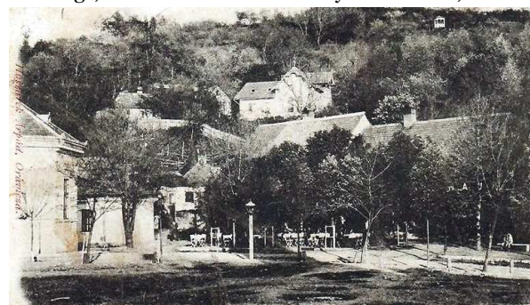
Fig. 20. Overview of the Shooting Garden (source: Urbanism Service, Oravița City Hall, online archive).
