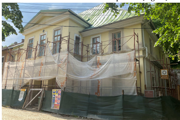
Fig. 12. Old theatre during restoration (July 2021) (source: Merciu G.).
