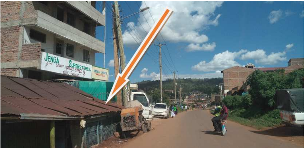
Fig. 8. A building (see the pointer) flouting the 6 metres building line in Mwembe.
