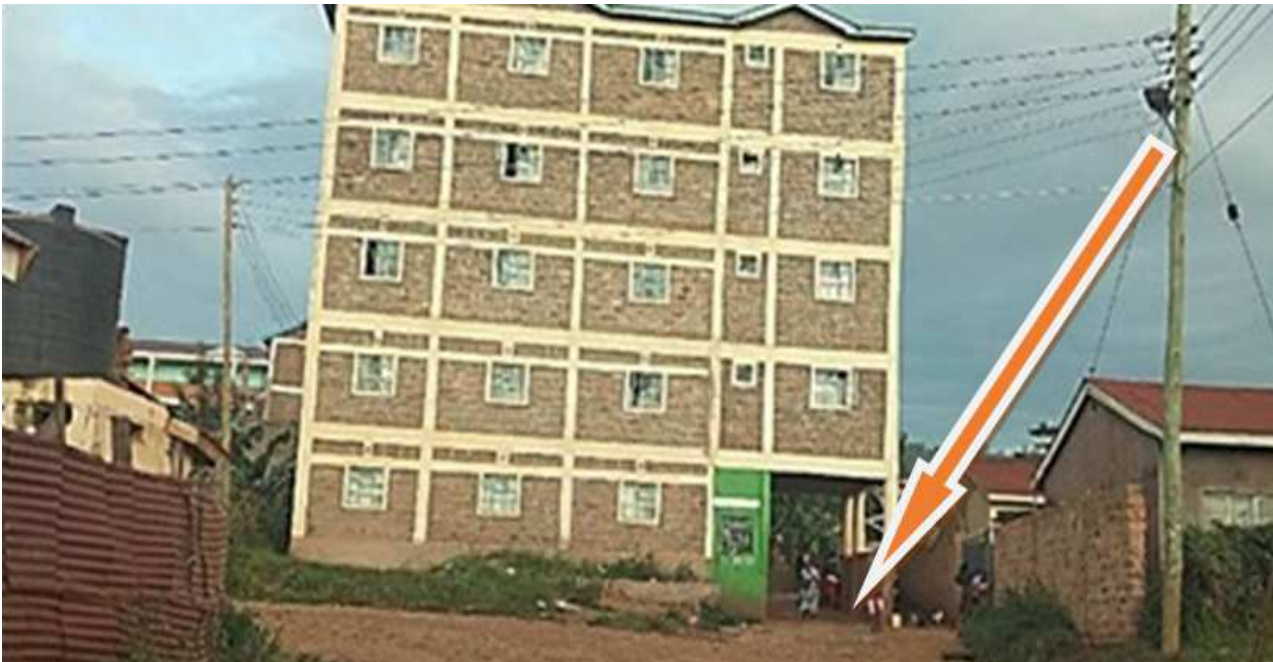
Fig. 6. A building (see the pointer) flouting the planning standard in Daraja Mbili.
