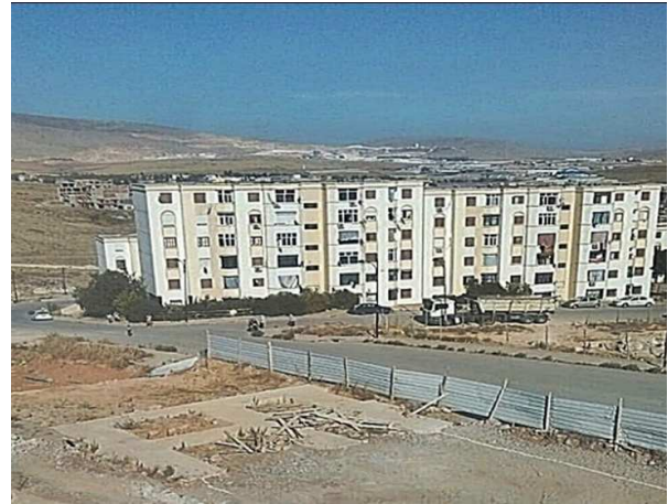
Fig. 10. Isolation and lack of bus stop in Massinissa (source: the authors , August 2019).
