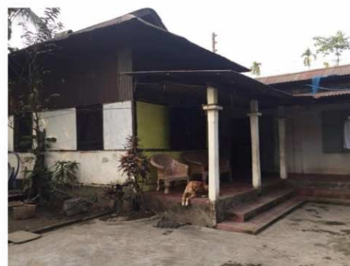
d) Post Lintel construction
