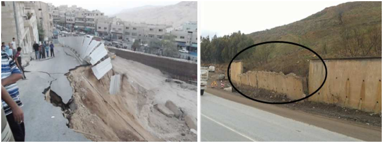
Fig. 6. Landslides in Médéa (2018).
