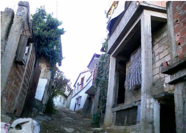
Fig. 9. Arbitrary construction in El-Afroun Municipality (source: the authors, November 4 th , 2016).
