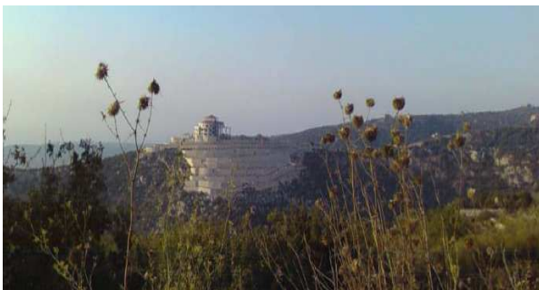
Fig. 3. Example of a personnel residential “reserve” under construction, dropped on a culminating hill, with stunning views over the sea and the mountains.
