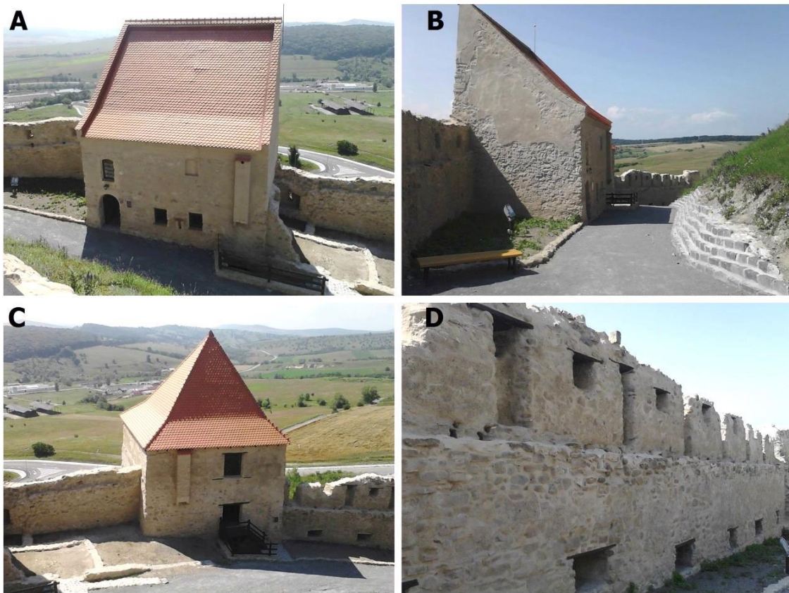
Figure 6: View over A, B – The Chapel, C – The Gresbig Tower or Scouts’ Tower and D – details on the wall between The Gresbig Tower and The Middle Fortress Gate after rehabilitation
