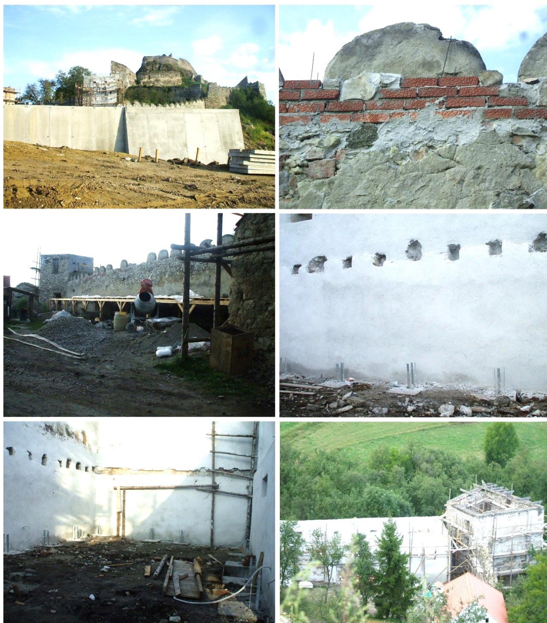
Figure 6: Details captured during rehabilitation (September 2010), underlining the invasive methods based on the extensive use of concrete in historical walls and foundations
